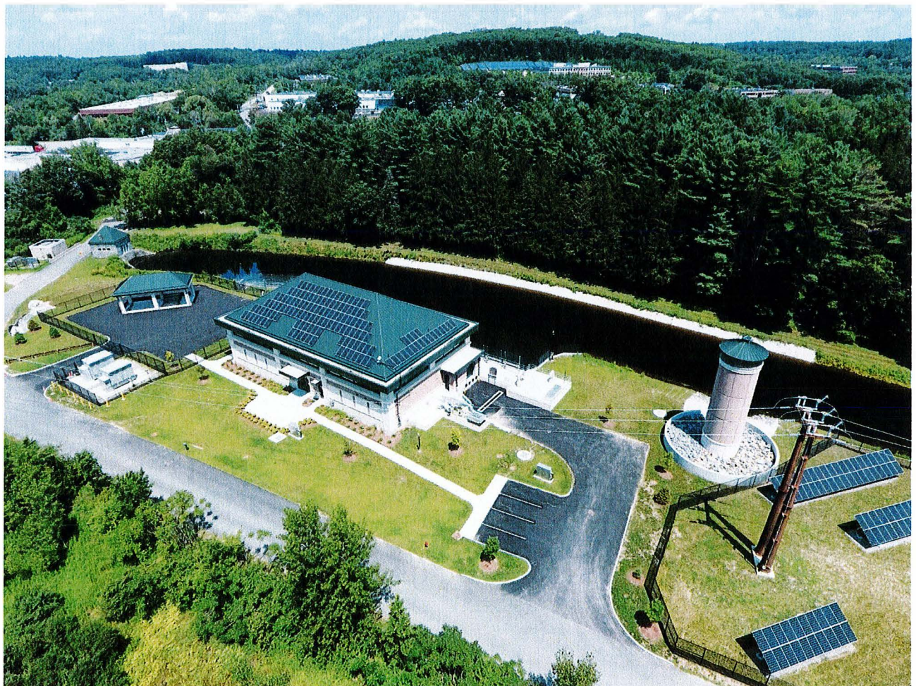
Wachusett Aqueduct Pumping Station
